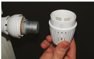
**3b)** In order to **lock** the adjustment range, position a limiter to the right of the number corresponding to the maximum desired opening and a limiter to the left of the number corresponding to the minimum desired opening. This prevents the head from being either opened or closed.
