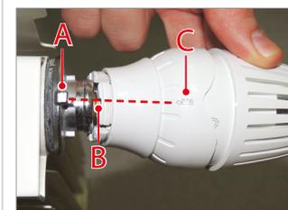
**2)** Connect the thermostatic head to the valve, making sure the valve pin (A), the small slot on the thermostatic head (B) and the Keymark symbol (C) are aligned.
