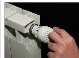
**4)** The head is now installed to the valve and can be moved to the required adjustment position by turning the knob.
