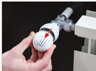
**1)** Turn the handwheel to position (3) and release it by pulling it forward.
